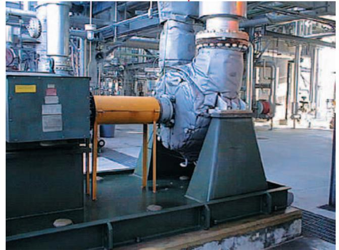
**Pump Packages** are provided to specifications and include lube oil piping, seal systems, monitoring instruments and drive train mounting. Pumps mounted with engine or turbine drivers and multiple pump modules are also available.
