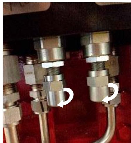
Fig 10.4 Flow regulator cap removal
