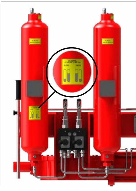
Fig 5.6 Example of Label Oil Level Application
